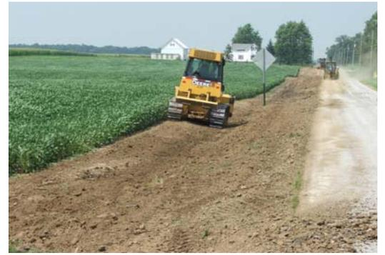
County crews constructed safety shoulders along a three mile section of Tri-township Road (above photo) for the St. Marys Township Trustees in anticipation of a pavement widening program in 2011. Additional easements were purchased, and the dirt from the newly constructed sideditches was moved to the edge of the pavement to create the wider shoulder.
