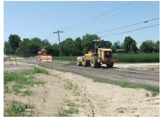
The Infirmary Road intersection to 25A (above photo) was reconstructed in order to provide a perpendicular approach and wider turn radii for school buses and semi-tractors. The existing asphalt was milled, placed and compacted in the new alignment and only a 3" mat of new finish hotmix was needed to provide a smooth driving surface. Special thanks to Mrs. Baranowski and the Steinke's for their cooperation in this much needed safety improvement.
