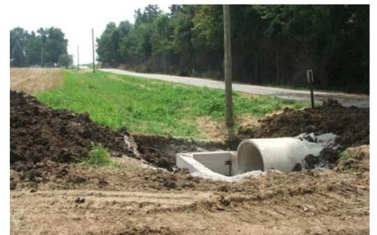
The above photo depicts a new elliptical concrete pipe crossing on Kettlersville Road with a concrete inlet drop box to allow stormwater to discharge into the pipe. The inlet is actually a section of a 3-sided box culvert (laid on its side) and cast by County crews at the garage.
