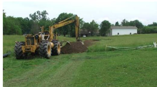
The Freeman Ditch is located two miles northeast of New Bremen. This subsurface tile drained a combination of agricultural and residential parcels. The project involved the installation of 225 feet of 30" and 1785 of 15" diameter tile (photo left). The \$ 39,657 project cost was assessed to the 143 acres benefitted within the watershed.
