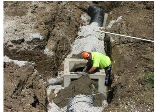
The photo above shows one of the 90 catch basin inlets installed during 2010. Holes are created, at a designed elevation in the sides of the precast concrete boxes to accommodate the stormwater pipe. Concrete is then mixed to mortar those connections to seal the new fitting. Such an installation allows stormwater traveling along the roadside to enter into the subsurface drainage tile.
