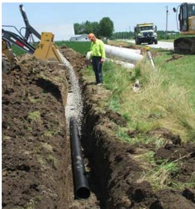
The photo to the left shows the replacement of century old storm tile with double walled plastic pipe. As noted above, a total of 2.74 miles of similar pipe was installed during 2010. Note on the photo that this new installation is placed outside the road right-of-way and on private property, away from the numerous buried utility lines in the highways easement.
