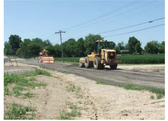
The Infirmary Road intersection to 25A (above photo) was reconstructed in order to provide a perpendicular approach and wider turn radii for school buses and semi-tractors. The existing asphalt was milled, placed and compacted in the new alignment and only a 3" mat of new finish hotmix was needed to provide a smooth driving surface. Special thanks to Mrs. Baranowski and the Steinke's for their cooperation in this much needed safety improvement.
