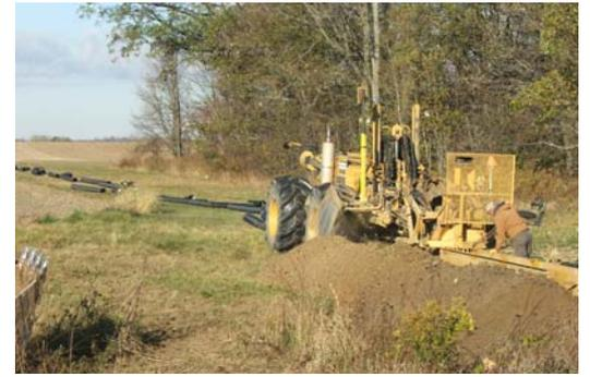
The Spencer Ditch # 2, located in Wayne Township consisted of the installation of 1590 feet of 10" and 1470' of 12" diameter subsurface polyethylene tile (above photo) plus one-sided construction of 1,425 feet of open channel. The \$47,265 improvement was assessed to the landowners in the 322 acre watershed.
