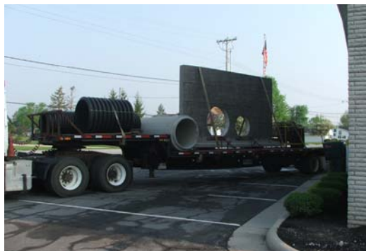
Included in the winter concrete casting operations are bridge beams, three sided boxes and precast headwalls. The photo above shows a pre-designed header/footer wall to be installed at the upper terminus of an open channel in Jackson Township.
