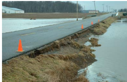
The above (left) photo shows the February floodwaters over County Road #25A north of Wapakoneta and flowing 20" deep through the Duchouquet Twp. House. The above right photo depicts the shoulder damage to the Bowsher Road north of the National Road in Logan Township.
