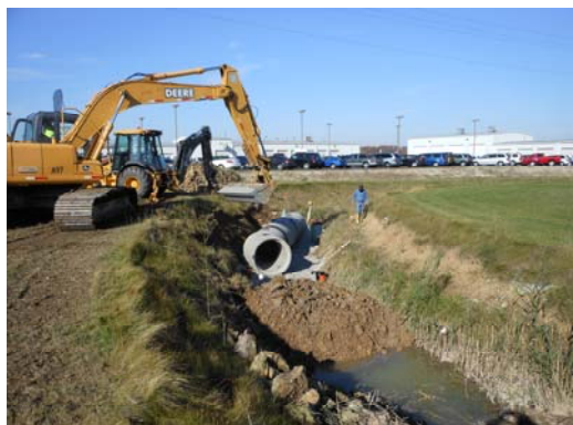
The Geiger Ditch is one of the County's permanent maintenance ditches and crosses diagonally through the Murotech manufacturing complex at the northeast corner of the City of St. Marys. Murotech is expanding their operations, in need of a second access across the ditch, and reimbursed the highway department for installation of the culvert for that driveway (below photo).
