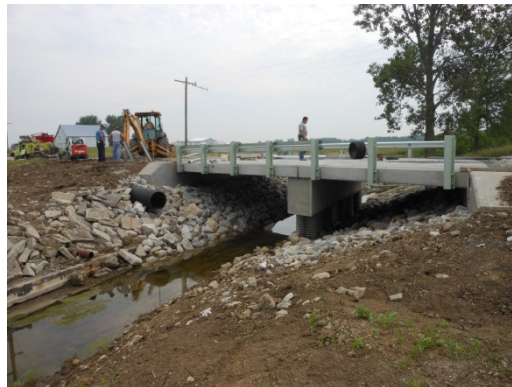
A two-span structure on Townline Kossuth was replaced using our forces and county manufactured precast concrete beams. The above photo shows the piling for the center pier in place and the redi-mix truck delivering concrete for the fabrication of the north abutment. The finished product (below) consists of two sets of beams 27' and 19' long, two new abutments and a center support pier with rip-rap placed preventing bank erosion. Total cost of this bridge, including the guardrail, approaches, and asphalt placement amounted to $92,000 or $ 74/sq. ft.. A recent study comparing county force account projects versus contracted projects using federal funds and guidelines found those project cost taxpayers over $160 per square foot.
