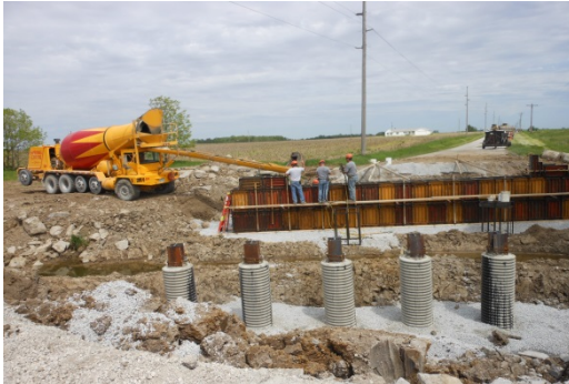
A two-span structure on Townline Kossuth was replaced using our forces and county manufactured precast concrete beams. The above photo shows the piling for the center pier in place and the redi-mix truck delivering concrete for the fabrication of the north abutment. The finished product (below) consists of two sets of beams 27' and 19' long, two new abutments and a center support pier with rip-rap placed preventing bank erosion. Total cost of this bridge, including the guardrail, approaches, and asphalt placement amounted to $92,000 or $ 74/sq. ft.. A recent study comparing county force account projects versus contracted projects using federal funds and guidelines found those project cost taxpayers over $160 per square foot.
