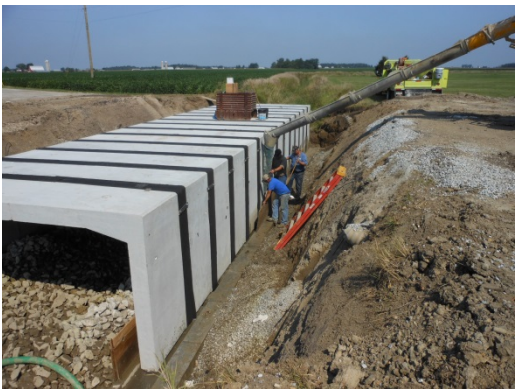
Seven smaller structures were replaced in 2013 using county manufactured concrete three-sided boxes. Since the program began in 1997, a total of 73 structures with 10 feet to 14 feet spans have been set. The upper left photo is a low profile 10' x 5' box with a poured concrete floor being placed on Townline Lima just north of the Fryburg East. This box along with one to the southeast on Fryburg East were installed in conjunction with the Huebner petitioned tile ditch project where landowners are having 5,700 feet of 18" and 24" diameter subsurface tile installed at an assessed cost to them of $179,853. Two 14' x 7' three-sided boxes were set on Winner Road just east of the Mercer County line. The upper right photo shows one of the boxes set on precast footers, waterproofing membranes placed on the joints and the crew grouting the sections into the footer.
