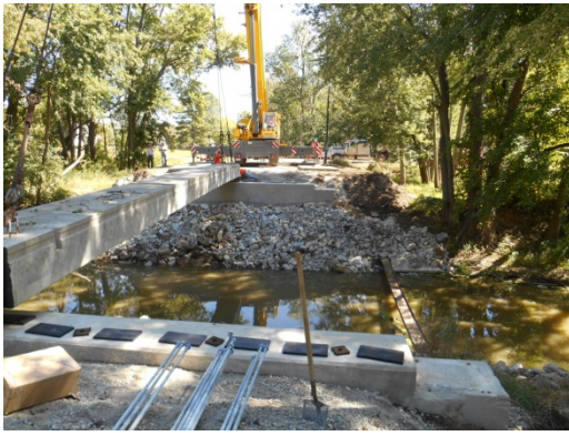
The above photo shows a crane setting 66' long concrete box beams on the bridge on the Salem Noble Road just 120' west of CR#66A. County crews removed the existing deteriorated deck and rehabilitated the abutments. A bid was let to purchase and set the beams and was partially financed by a 0% 20 year loan from the Ohio Public Works Commission. This 66' long by 28' wide deck cost just over $100,000. In 2002, a similar box beam deck on Greenville Road was 72' in length and 32' in width was purchased for $57,000.
