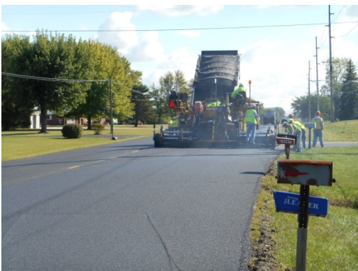
33A Paving (above) showing half of the roadway (15’) being resurfaced in one pass.
