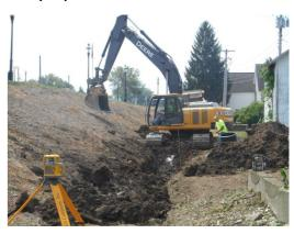
In order to fill some of the funding gap, our staff was "hired" by the Village of New Bremen in 2014 to install storm sewers at two different locations along with the placement of 1006 tons of rip-rap for erosion control of the drainage channel. The above photo shows the replacing of 530' of a substandard storm sewer just west of SR#66. The below photo is the installation of 528' of storm sewer with manholes in the Bunker Hill Industrial Park west of town.
