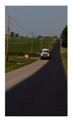
CHIP AND SEAL PROGRAM: This maintenance practice can extend the life of a pavement 8-10 years by applying a layer of liquid asphalt followed by a layer of #8 limestone A total of 23 miles were full sealed with an additional 22.5 miles strip sealed. A total of 164,300 gallons of liquid asphalt and 5,525 tons of stone were applied in the program with a material cost of \$360,845. The follow up fog seal application with 28,700 gallons of liquid asphalt had a material cost of \$41,627.
