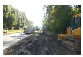
County crews installed storm sewers in the sideditches of Amsterdam Road east of SR# 66 (above photo) and then placed several hundred yards of dirt in order to build safety shoulders and eliminate the steep sideditch slopes. Special THANKS to Crown Control for purchasing the piping necessary to enclose the ditch along their property.
