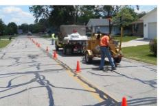
ROADSIDE DRAINAGE: In the ongoing effort to replace century old deteriorated storm sewers, crews in 2014 installed 390 feet of reinforced concrete pipe through the roadway, 8,305 feet of smooth walled polyethylene plastic pipe within the road right-of-way along with placement of 75 new catch basins to provide for surface water inlets to the pipe.
