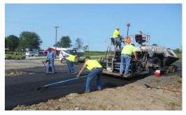
The above photo shows our crews placing hotmix over the 25A box culvert replacement. Having the paver and rollers allows us to open the roadways soon after the bridge/culvert installation and not wait for scheduling with independent contractors. In 2014 our employees placed 832 tons of hotmix on numerous bridge/culvert and safety improvements.
