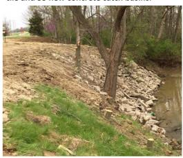
Koop Creek travels extremely close to and parallel to CR#66A just south of SR#219 and had severely eroded the stream bank near the edge of the pavement. Crews worked with nearby farmers who had demolished several concrete silos by hauling the broken concrete to this site to reconstruct the eroded bank (above photo) and provide a wider safety shoulder for CR#66A. Rip-rap from a stone quarry would have cost \$18/ton.
