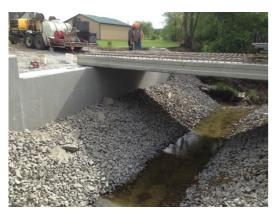
The bridge on Santa Fe Line Road north of Fairmont Road was fully reconstructed using 31' long county manufactured precast concrete floor beams. Existing abutments were nearly a century old and had structural issues. A hydraulic demolition hammer was used to remove the walls which were then used for erosion control along the stream. The new abutments rest on a series of 10" steel piling driven an average of 25 feet below the flow-line of the stream.
