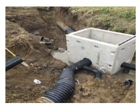
The above photo is a concrete storm-water basin cast by county crews showing multiple drainage tile hookups. As an ongoing program to improve drainage within the road right-of-ways, in 2015 employees installed 628 feet of reinforced concrete pipe, 11,500 feet of smooth walled polyethylene tile and 55 new concrete catch basins.
