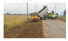
The Washington Township Trustees hired county crews to widen and provide safety shoulders on Kettlersville Road south of SR#219. The dirt needed for the widening came from a nearby pond excavation.
