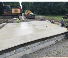
Above left photo shows 32' long county manufactured beams on Wrestle Creek Road prior to the placement of a 6" deep concrete poured deck. Upper right photo shows the county crews placing a similar 6" deck over 27' long county beams on the Heitkamp Road. This 6" extra depth provides for a total beam depth of 20" and the needed load carrying capacity for today's highway loadings.
