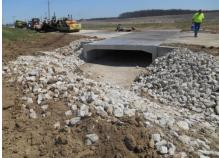
The above photos are two of the three sided box installations manufactured and installed by the county crews. The left photo is on the Thrush Ditch that drains five hundred acres and thus requires 7' deep legs to provide the needed capacity. Upper right photo on the Swartz Road is a similar box with just 5' legs (three foot opening) and a concrete floor due to a much smaller 100 acre watershed.
