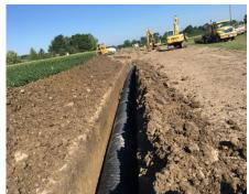
PETITIONED DITCH PROJECTS: Two projects petitioned through the Commissioners and designed and inspected by this department were the Fisher #2 and the Blasé #2. The Fisher #2 in Salem Township (upper left) included the installation of 1000 feet of 24" diameter seal plastic tile through a wooded area and 800 feet of open channel at its outlet at an assessed cost of \$ 38,000.
