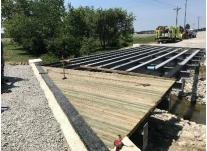
Upper left photo shows county manufactured 33' long beams being set on the Hardin County line. Once placed, a 6" deep concrete deck is poured to lock the beams together and provide the necessary carrying capacity for a 33' long span. Special thanks to the Hardin County Engineer for sharing the cost.
