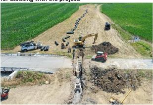
The Accuntius Joint County ditch with Shelby County replaced a failed clay tile originally installed in 1904. The photo to the left shows the contractor crossing Winemiller road and the 24" diameter tile strung out for placement with a trencher. This 2.9-mile tile project was by far the
