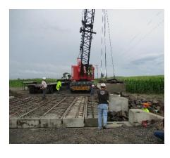
Photo left shows the bridge crew setting the 26' long precast county beams (cast in February) on the Auglaize Hardin County line. Nine beams will provide for a 27' wide deck. Thanks to Mike Smith, Hardin County Engineer for assisting with the cost of this structure.
