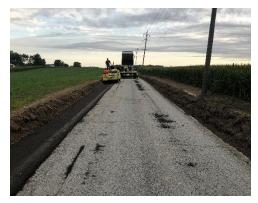
Along with County roadway projects, the department widened a half mile of Enneking Road for the Jackson Township Trustees. Recycled asphalt grindings were placed 8" deep and two feet wide on each side of the existing pavement (left photo) and compacted to transform a 16' wide pavement to 20'. Material cost of the grindings used was at \$10/ton versus new base hotmix at \$75/ton.
