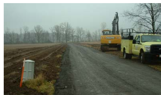
The Logan Township Trustees hired County crews to extend Kossuth Loop Road using 820 tons of milled asphalt grindings.
