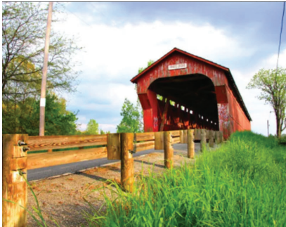
Swartz Bridge, Wyandot County, Ohio
