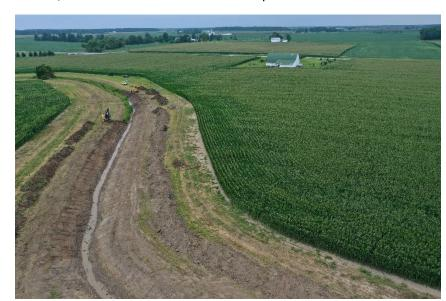
The Sheipline Ditch in Duchouquet Township began construction in the summer of 2022 but is not yet complete. The remaining construction items include boring under the CSX rail line and installing the remaining 1,200 feet of tile upstream of the railroad. The work is being performed by Liebrecht Excavating.
