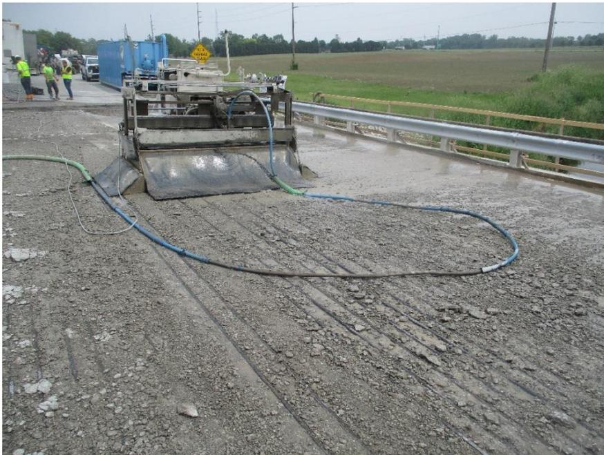
washer that sprays water at **15,000+ psi** to break up the bad concrete, leaving the solid concrete in place. After the old concrete was removed a new concrete deck was poured in place to complete the project. The final project cost came to \$176,057.18 and was paid out of our dedicated road and bridge funds.
